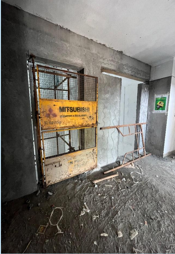
T1 SERVICE LIFT ERECTION
