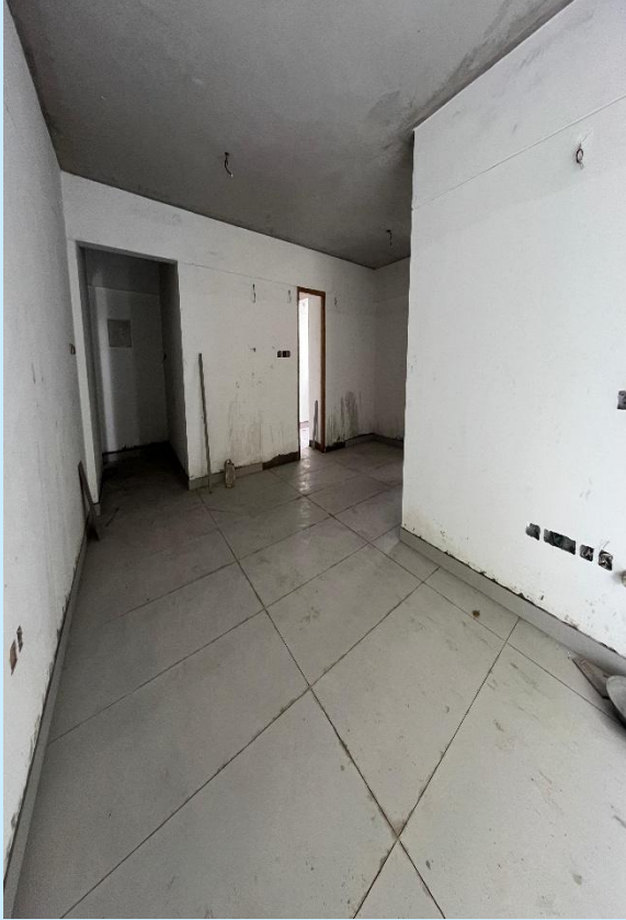
T1 3 RD FLOORING WORK
