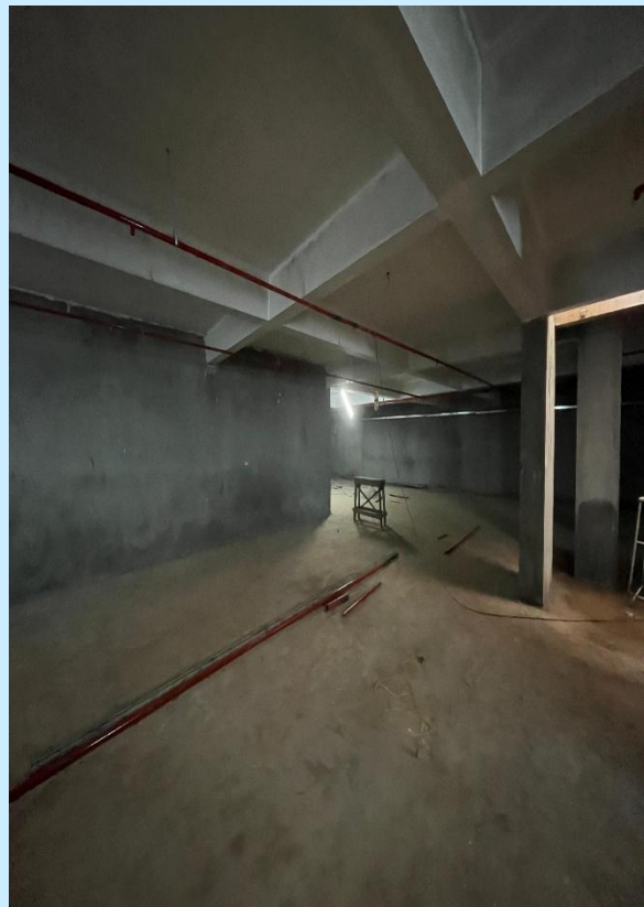
T1 B.F FIRE&SAFETY WORK
