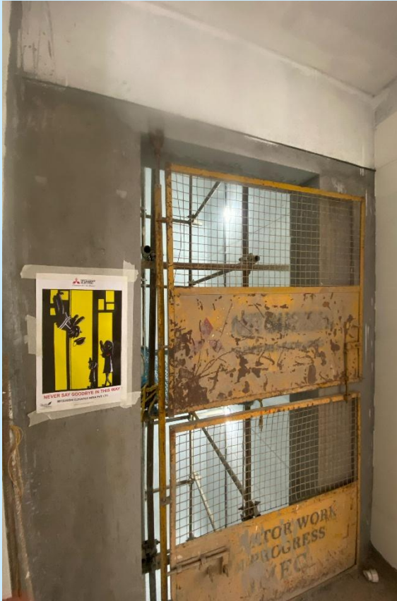
T2 LIFT ERECTION
