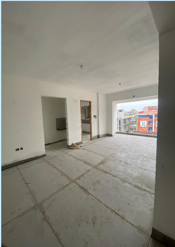
T2 4 TH FLOORING WORK
