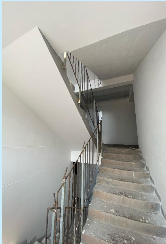
T2 MAIN STAIR PUTTY WORK
