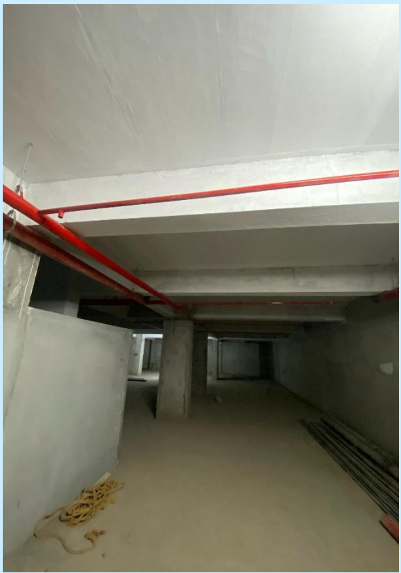
T2 B.F FIRE&SAFETY WORK
