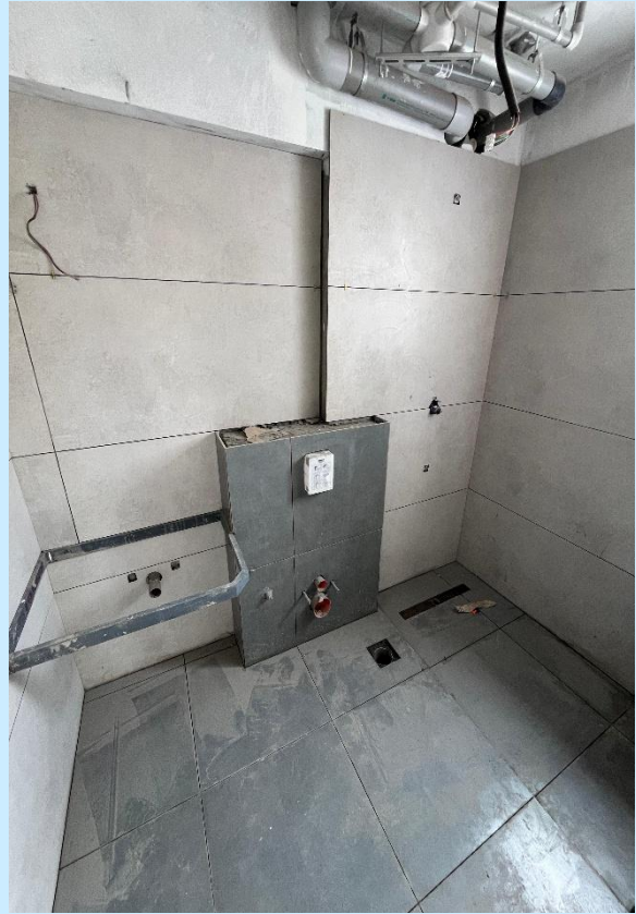
T1 3 RD TOILET TILE WORK
