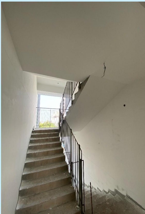
T2 FIRE STAIR PUTTY WORK
