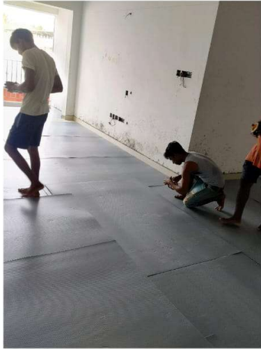
Joint filling & floor protection
